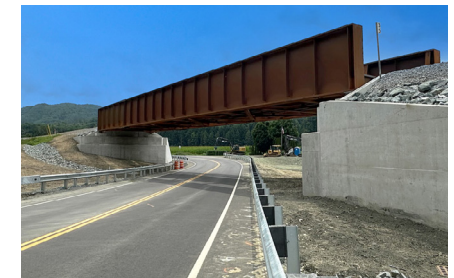
Royalton Completed Bridge View.
