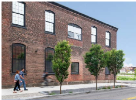
PINE STREET TRANSIT-ORIENTED DEVELOPMENT DISTRICT MOBILITY AND GREEN INFRASTRUCTURE IMPROVEMENTS, PAWTUCKET, RI
